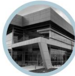
DATA CENTER - PRIVATE CLOUD
